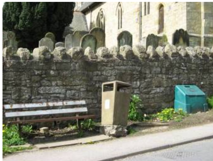
Thought could be given to co-ordinating some of the utility items in the street
