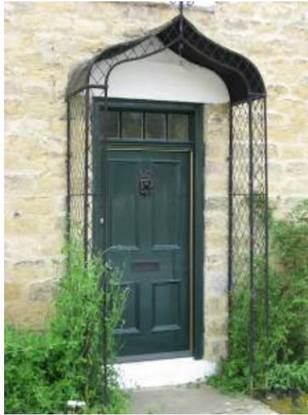
A beautiful example of a solid panelled door with fanlight over and an unusual lattice ogee topped porch
